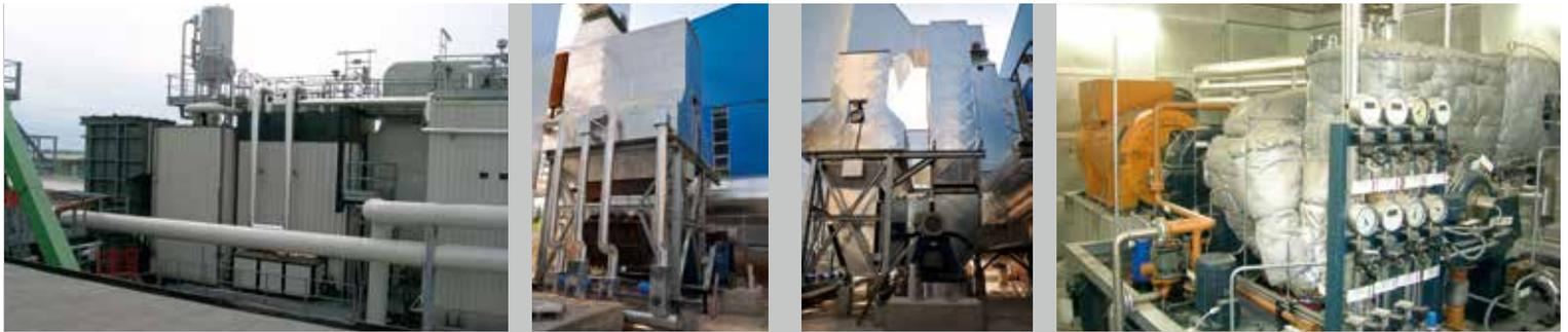
Area Impianti's solutions covers a wide range of systems, such as air heating through fumes/air heat exchangers and steam generation with boilers. Steam is then used for process needs and/or electricity production in a turbine. When the fumes temperatures is below 600°C, an interesting alternative
