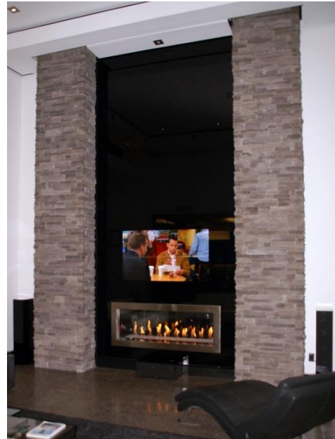
Vanceva Absolute Black interlayer with a clear window cutout for television - 2235 mm x 4775 mm - 88" X 188"
