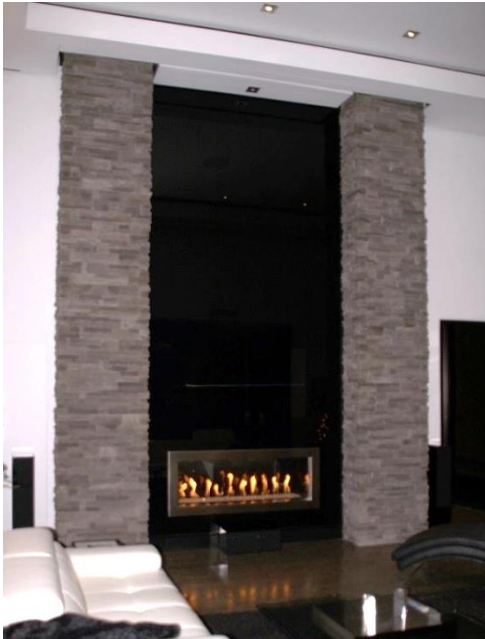
Vanceva Absolute Black interlayer with a clear window cutout for television - 2235 mm x 4775 mm - 88" X 188"
