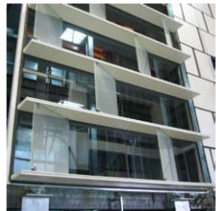
Figure 9: Façade mock-up of Star Place facade
